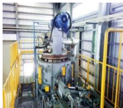
Two microwave activation furnaces
